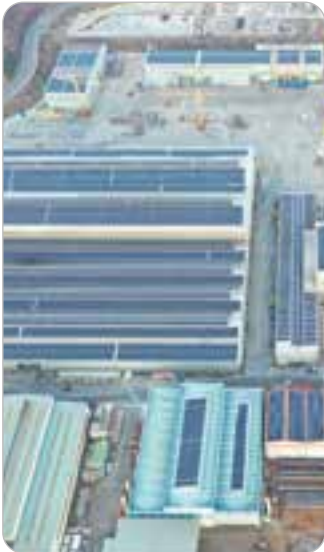
Seongdong Project Korea | 20MW | 2022
