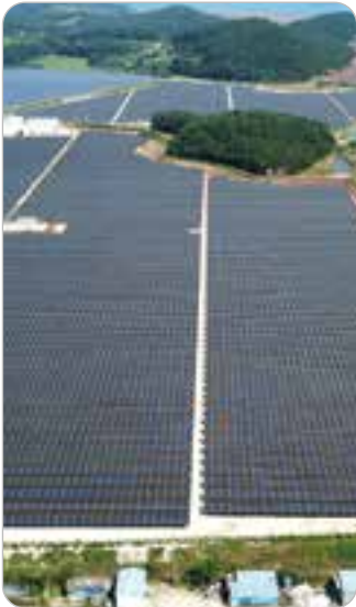
Samyang Project Korea | 17MW | 2020
