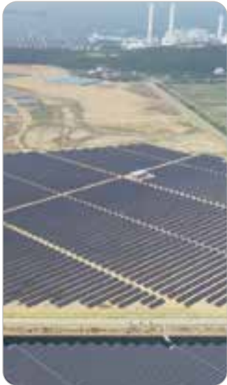
Dangjin Project Korea | 25MW | 2020
