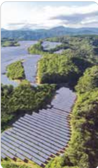
Tojo Project Japan | 33MW | 2015
