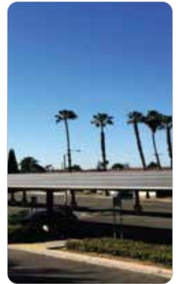
School Project USA | 3.3MW | 2013
