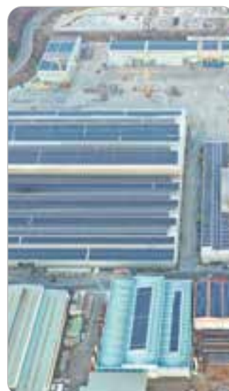
Seongdong Project Korea | 20MW | 2022
